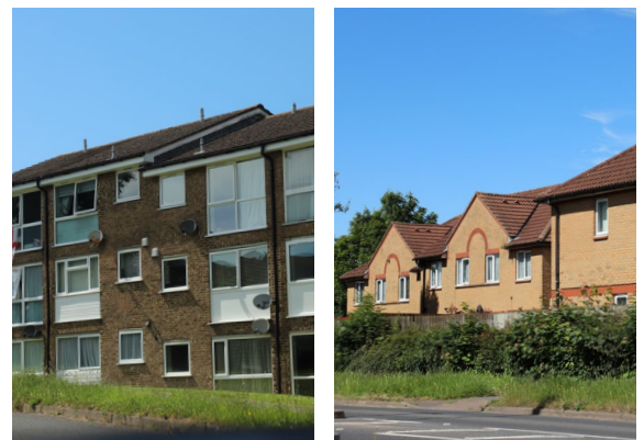
Fig 02.19 Typical residential character
