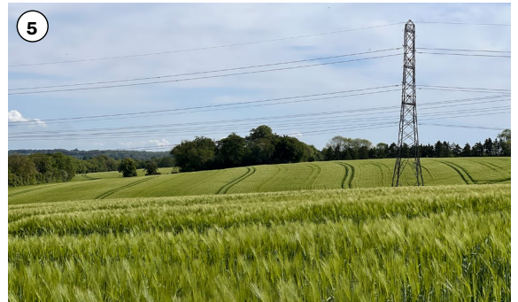
Fig 03.6 H2 open fields, sloping topography and NGET overhead power lines in the north
