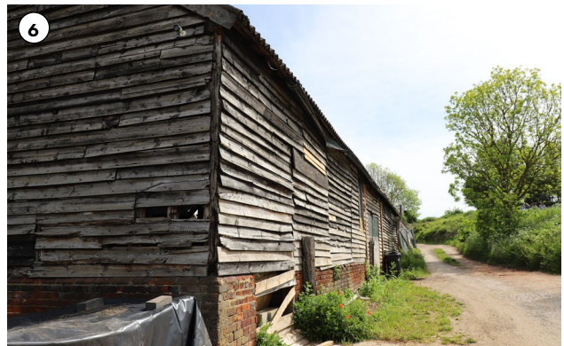
Fig 03.55 Listed Wood End Farm Barn
