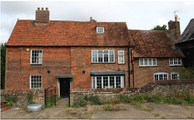
Fig 03.40 Wood End Farmhouse
