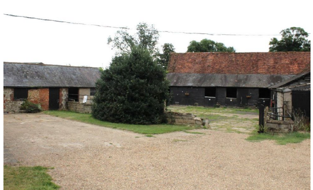
Fig 03.45 Westwick Row Farm courtyard
