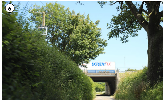
Fig 03.61 Hogg End Lane as it traverses under the M1
