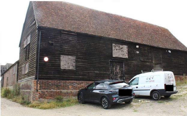
Fig 03.42 Large Barn at Wood End Farm
