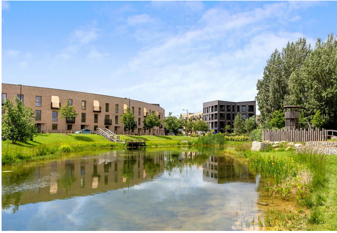
Integrated attenuation features, Barton Park
