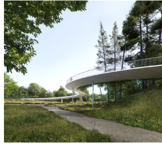
Footbridge over N10, France
