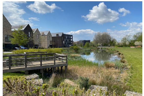
Attenuation ponds with permanent standing water | Barton Park, Oxford
