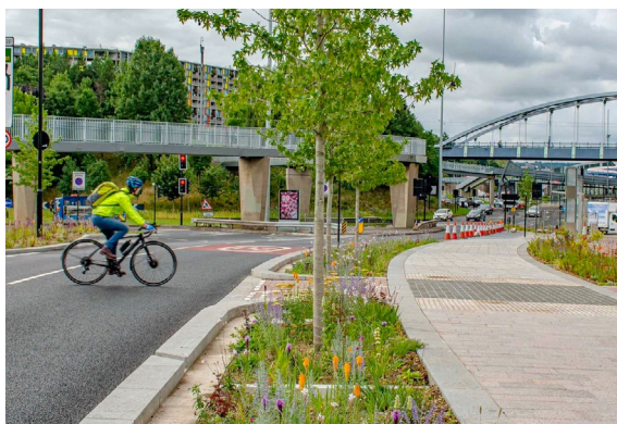
Roadside rain gardens
