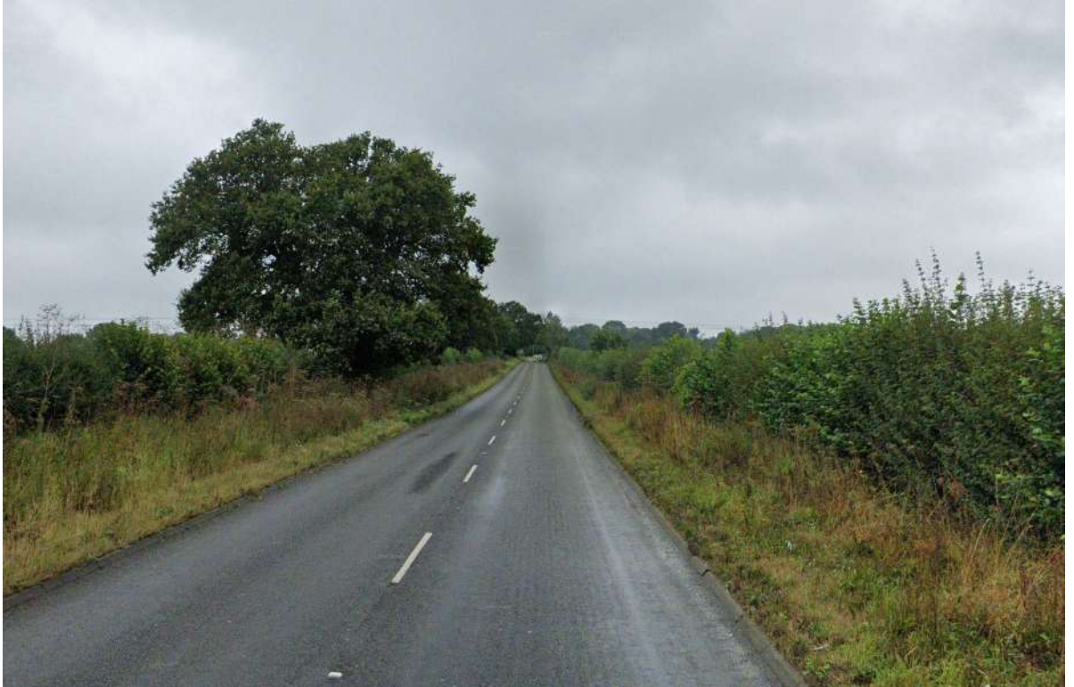
Fig 08.4 Existing view looking west on the B487
