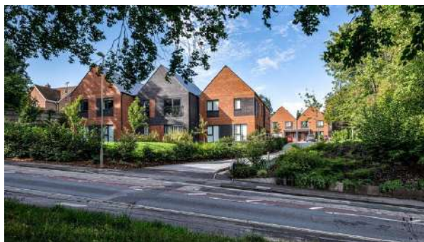
Setback residential frontage with filtered views | Fairlinch Close, Winchester
