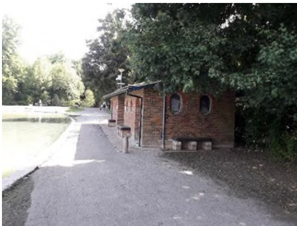
Closed Causeway toilets
