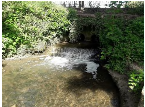
Outflow from lake back into River Ver
