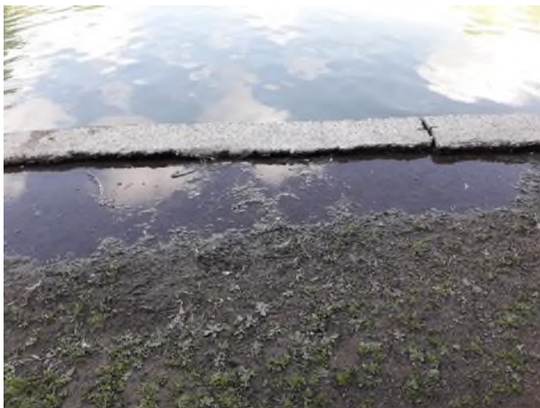
Concrete edging to the lake
