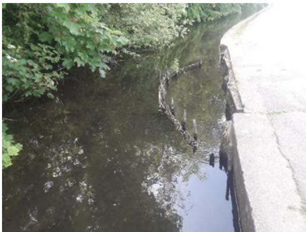
Sluice from River Ver feeding the lake
