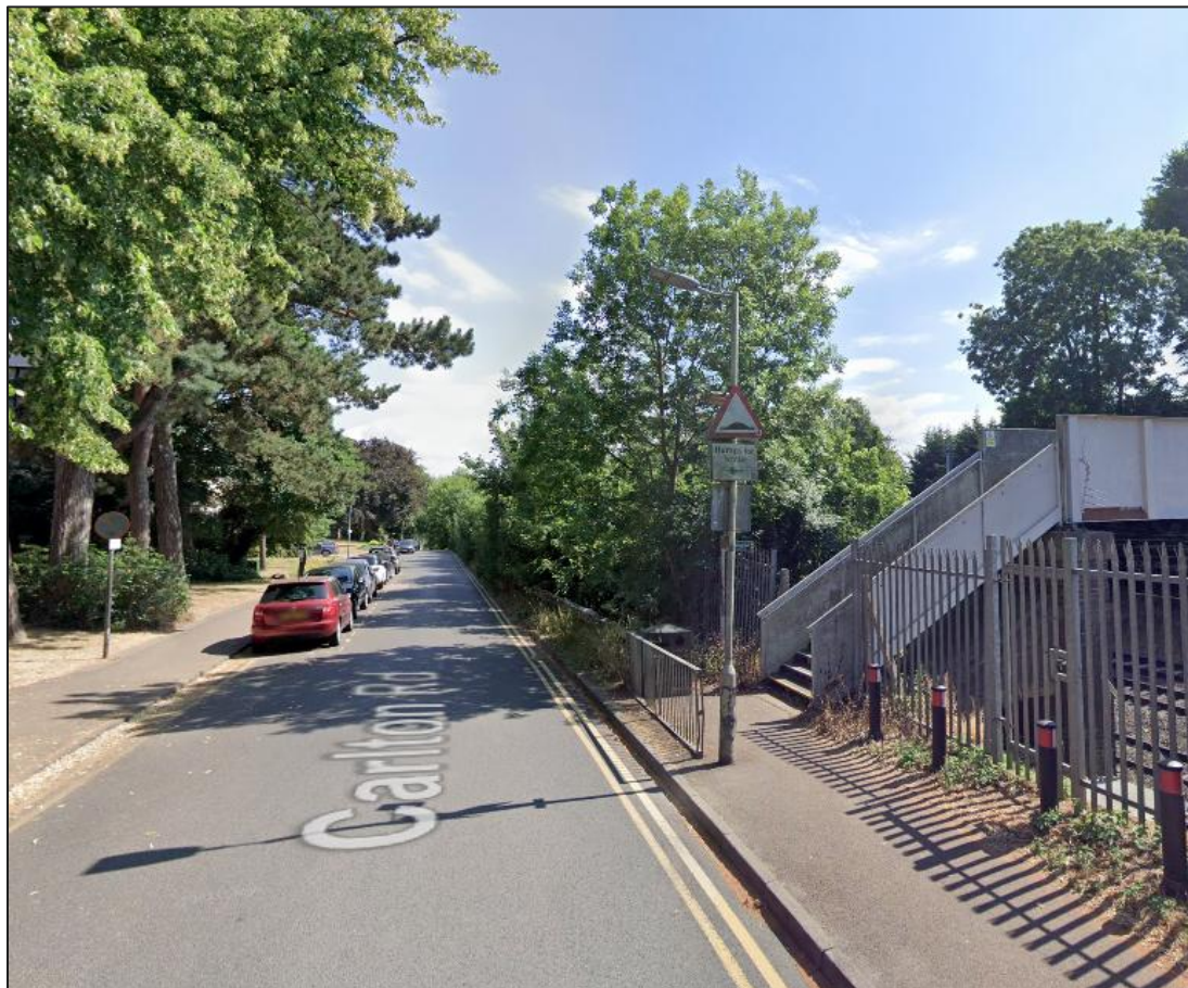
Photograph 2.9: Footbridge Between Carlton Road and Footpath 19
