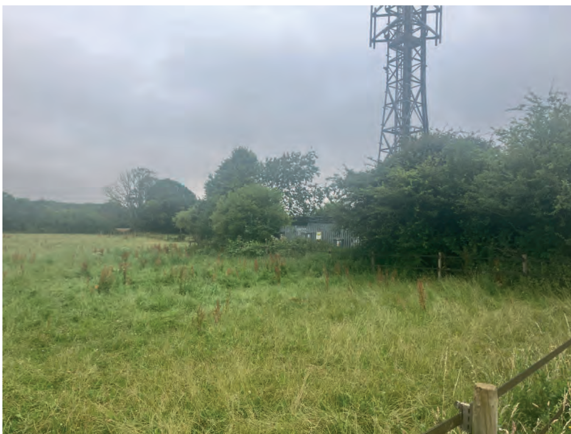
Plate 4: View looking at mobile phone mast within the central part of the site
