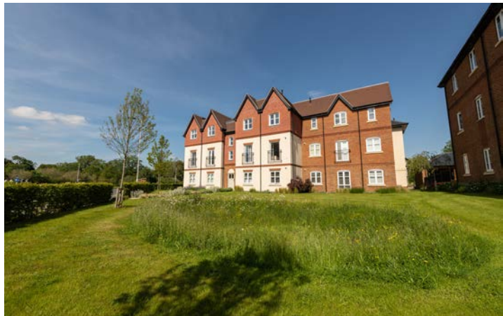
Example of a dry infiltration basin alongside residential development, Woodhurst Park, Berkshire
