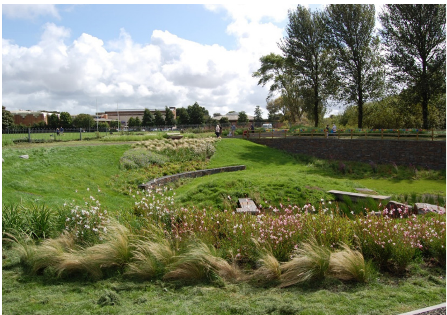
Example of Llanelli Rainscape - Shallow basins, filled with swathes of plants, catch and clean the surface water runoff before soaking into the ground
