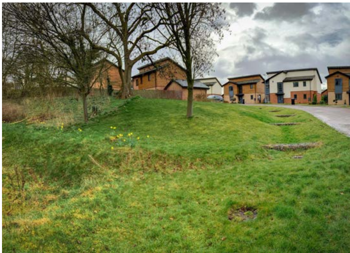
Example of an edge of parkland swale going downhill, featuring check dams to slow the flow
