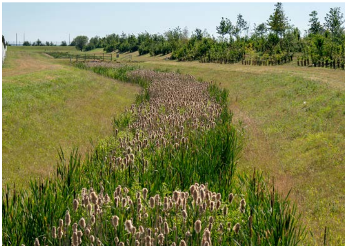
Example of a vegetated linear parkland swale, planted with wetland grasses
