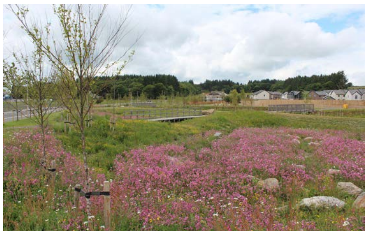
Example of planted SuDS basin in Countesswells, Aberdeen
