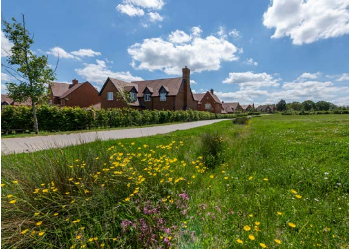
Example of an edge of parkland swale, planted with wetland grasses & plug planting - managed to be naturalistic as part of the overall parkland setting
