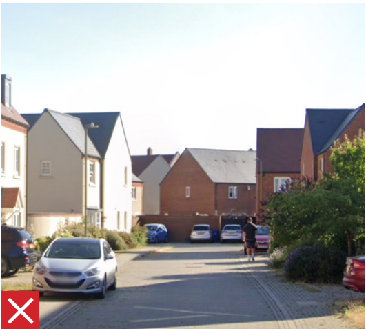
Car parking and boundary wall
