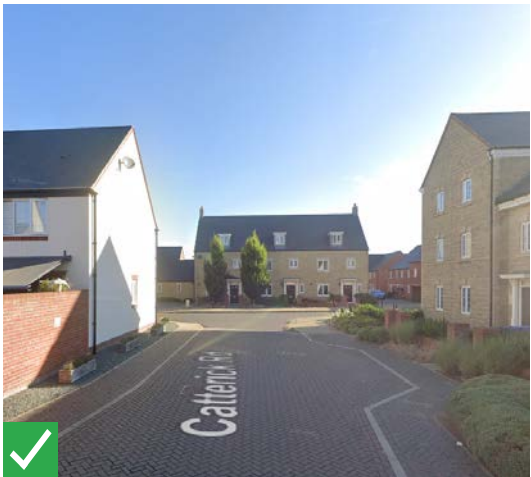
2.5 storey terrace successfully terminating vista
