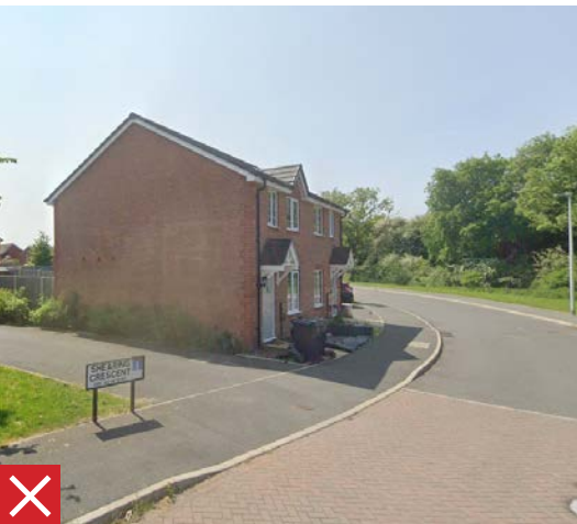
No windows to street or POS opposite
