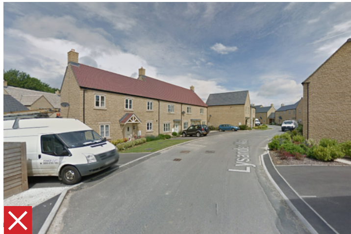
Blank gables interrupting building line flow
