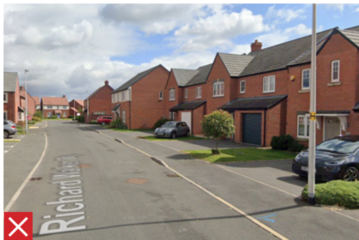
Building line interrupted to accommodate parking
