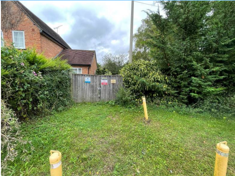
5. Lower Luton Road, sewage pumping station.
