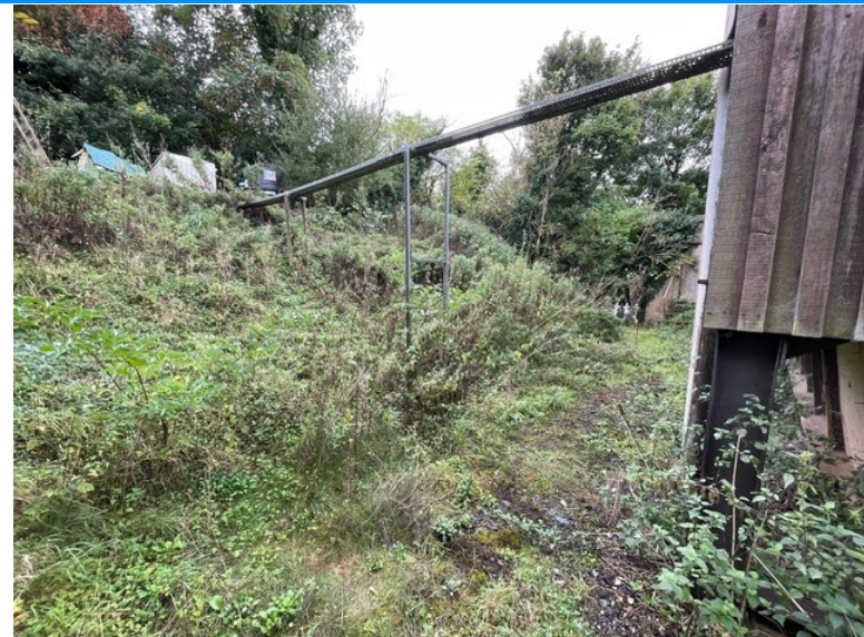
24. Rear of indoor arena, showing cut and level difference.
