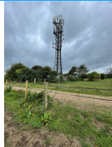
64. The communications mast adjacent to the main farm track.
