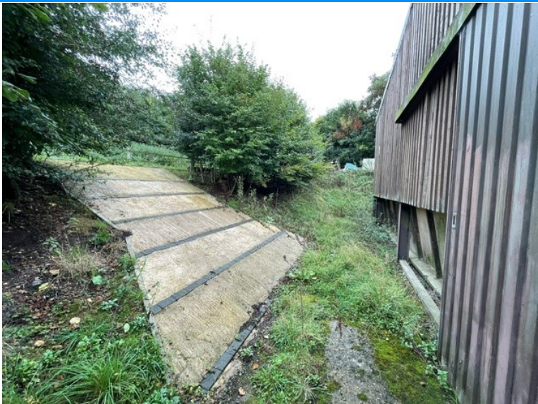
23. Access down from track to indoor arena – showing change in levels (and cut).
