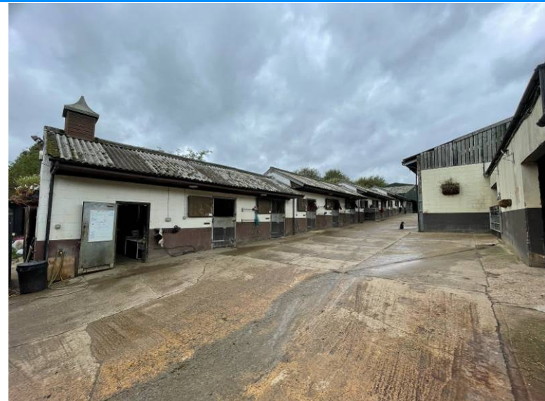
8. Southern end of the stable block – looking north.
