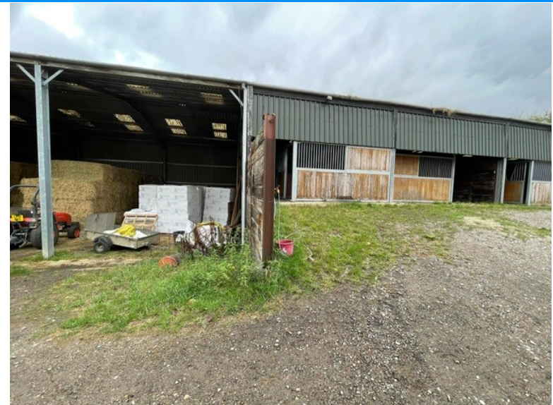
26. Showing change in levels & retain between the loose horse housing and barn.
