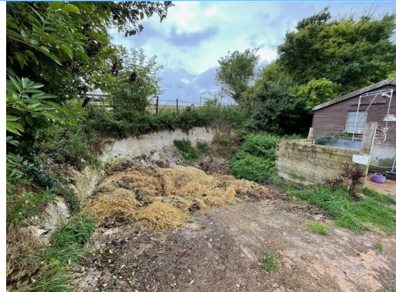
34. Existing cut into hill, showing chalk face.
