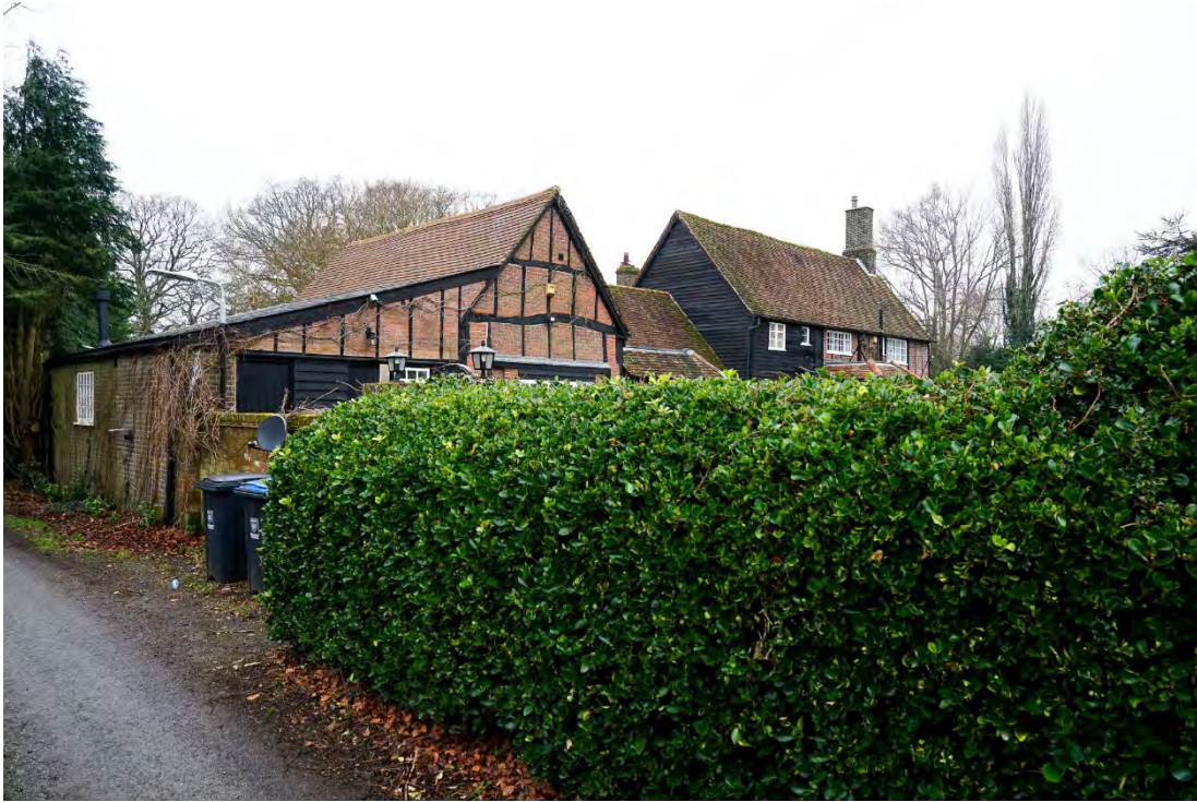
Plate 15: East elevation of Holtsmere Manor and its outbuildings
