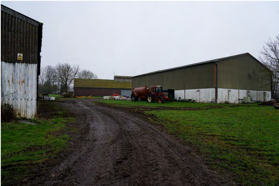
Plate 22: Agricultural sheds at Great Revel End Farm, facing north towards the farmhouse (screened)
