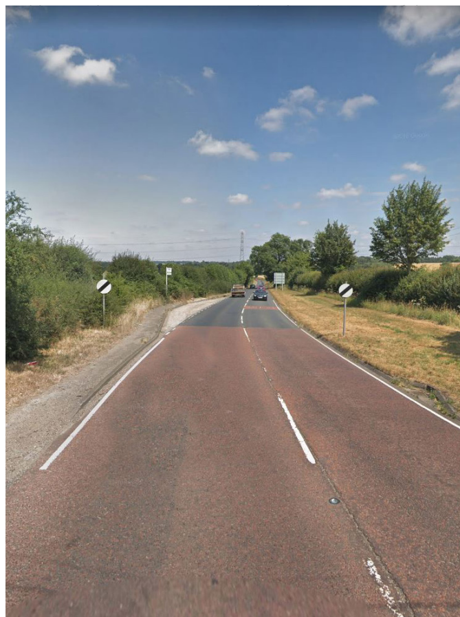
Redbourn/Hemel Hempstead Road (B487)
