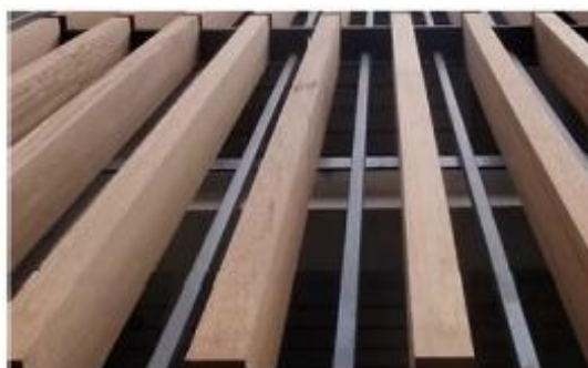
Figure 3 - Solar shading devices (example)
