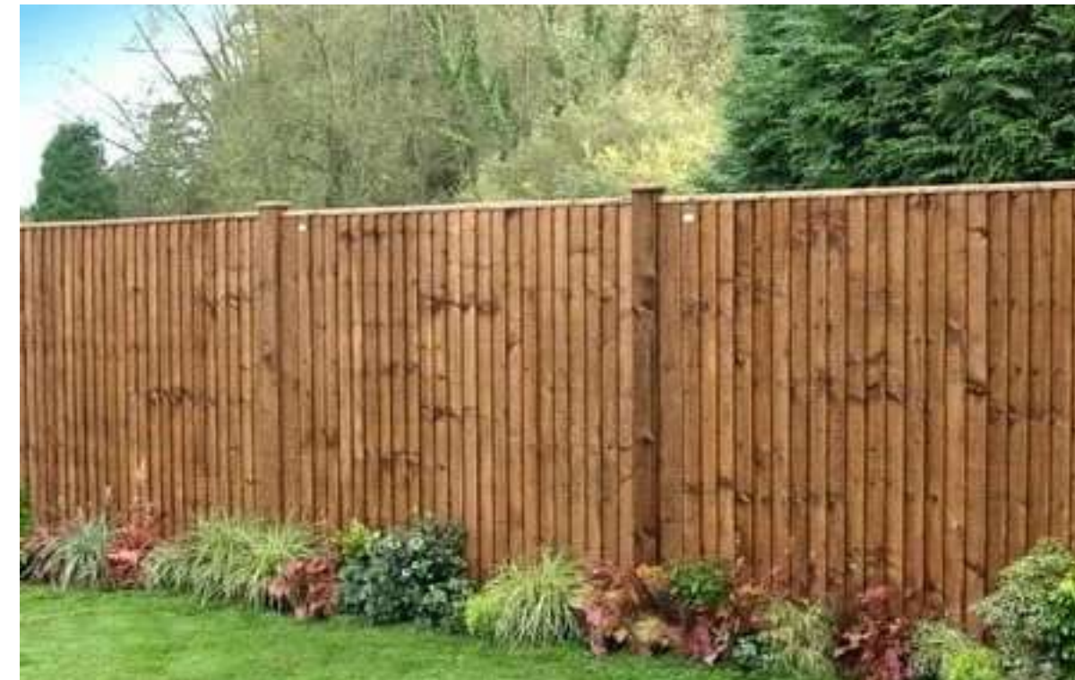
Close boarded timber fence
