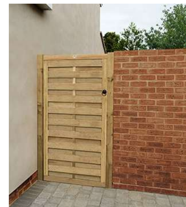
Brick wall with timber gate
