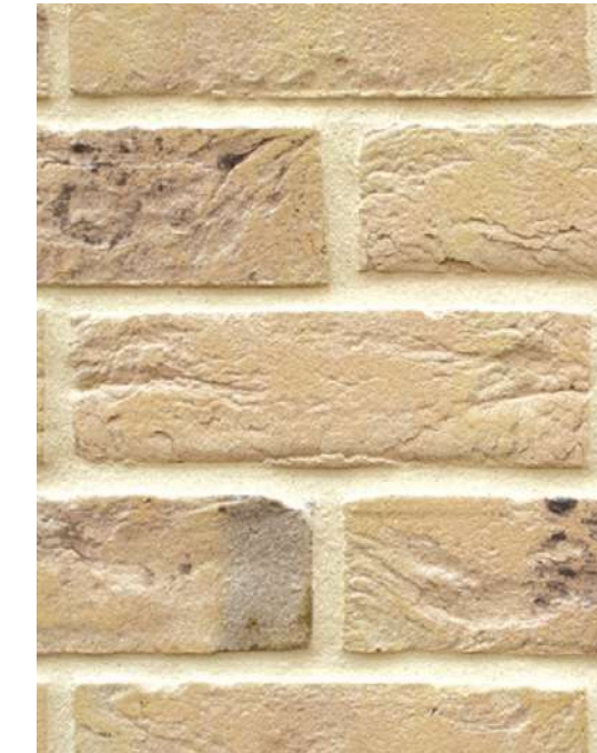
Buff brick with light mortar
