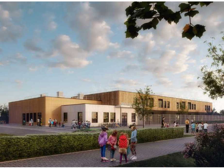
HLM Architects - Abbey Farm Primary School
