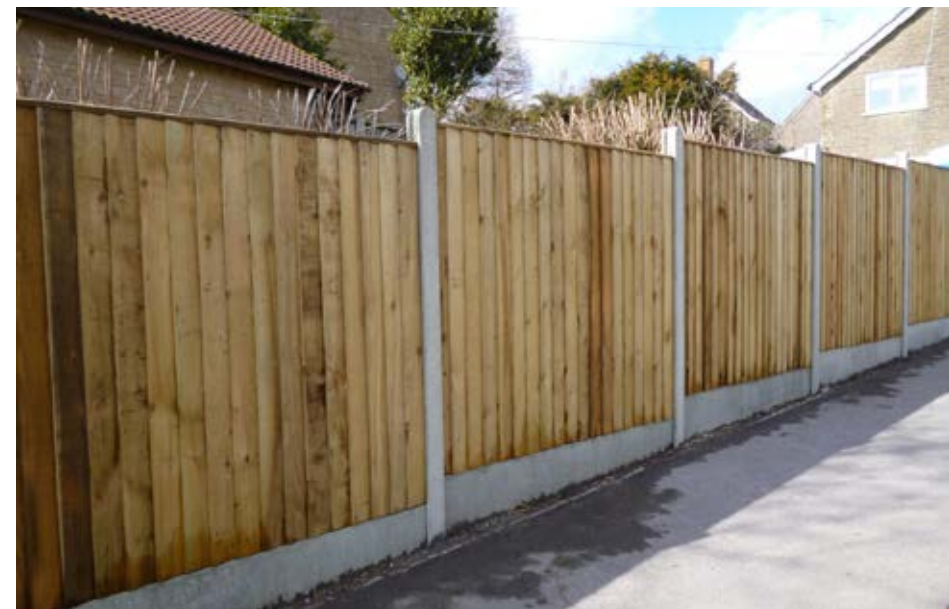
Figure 117. Example of low concrete wall with close boarded fence in road incline
