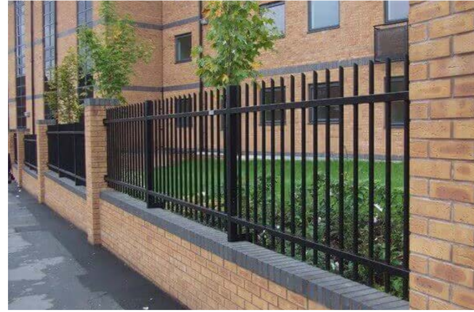
Figure 115. Example of low brick wall with railings
