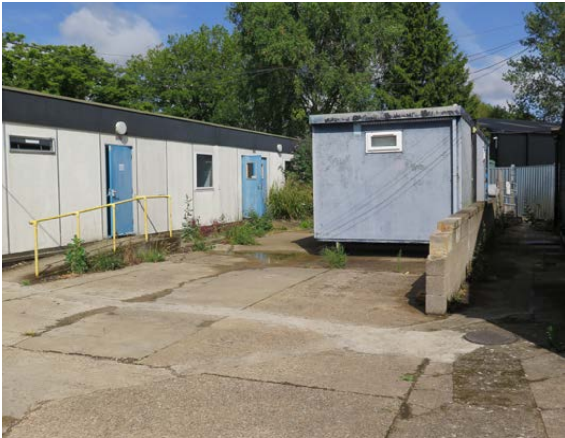
Staff temporary offices
