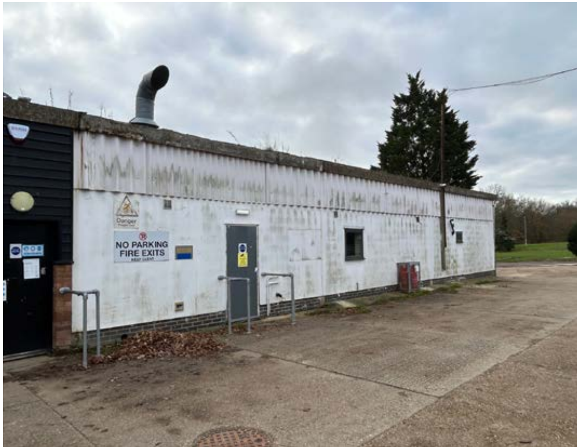
Gas Installation Building
