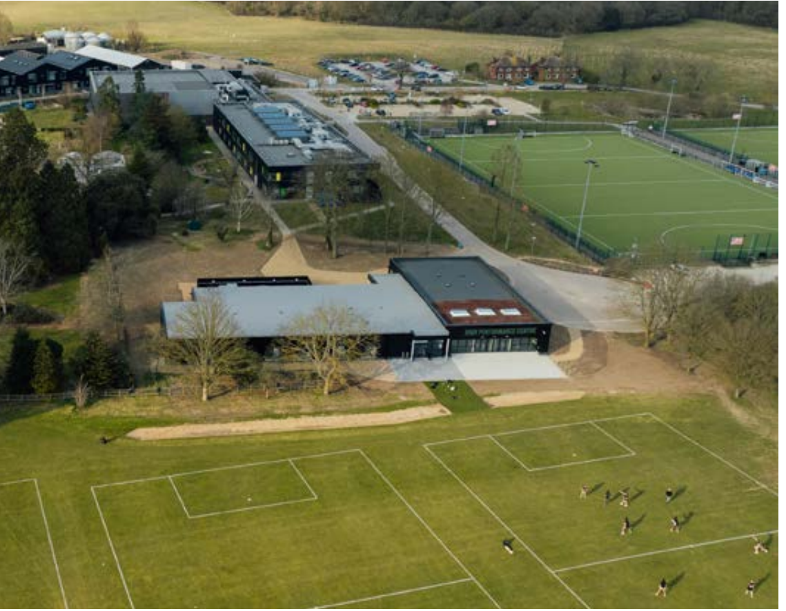
Discovery Centre & High Performance | Sports Pavilion
