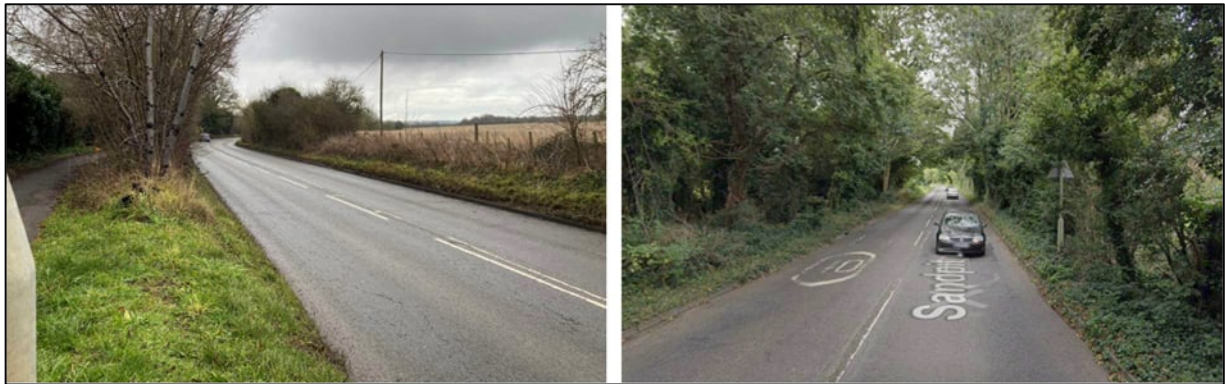
Figure 20 – Sandpit Lane Carriageway Conditions
