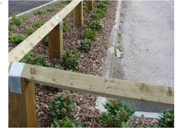
Example of timber knee rail fence
