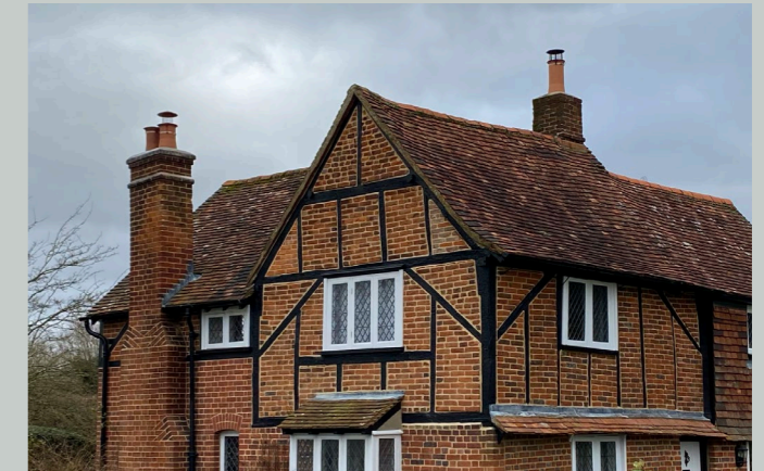
Tall chimney stacks
