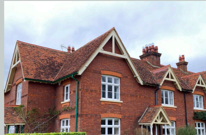
Gable forms with timber detailing
